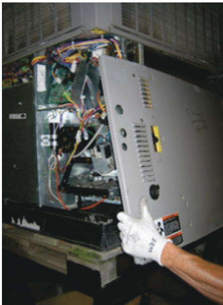
Fig. 34 – Replacing Right Side Panel
