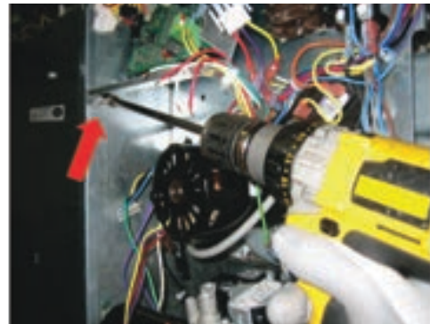
Fig. 31 – Removing Screw Under Control Board Panel A210078
